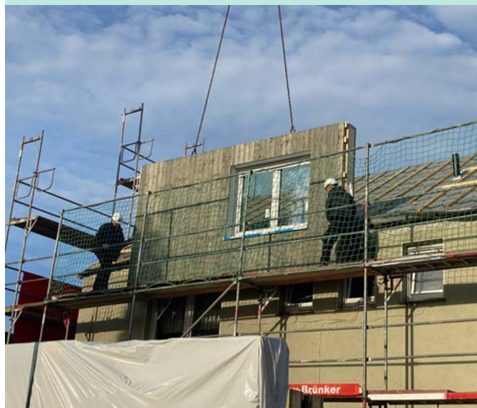
The use of 2D timber construction modules provides strong opportunities for the serial energetic refurbishment of e.g. apartment buildings in Germany
