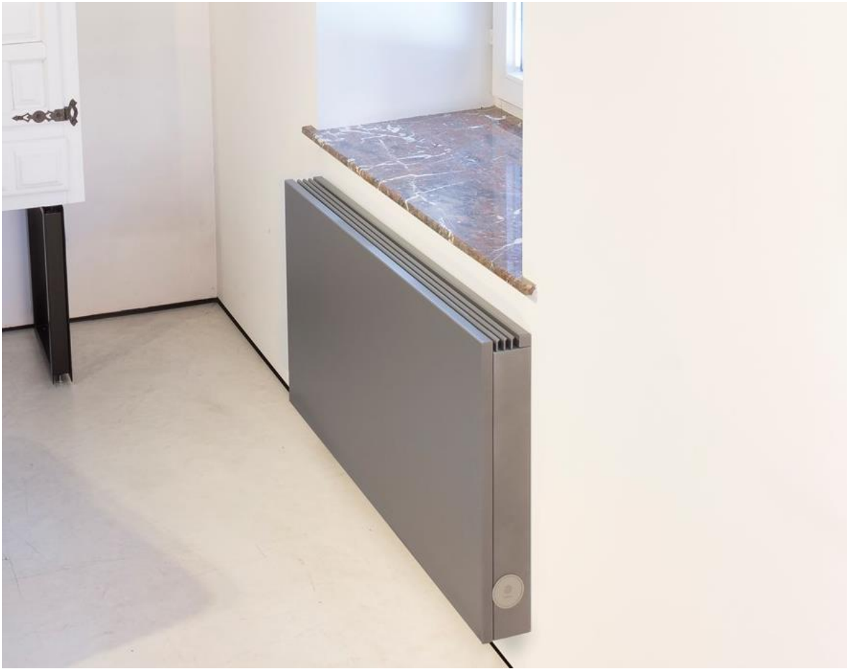
Figure 19. Example of an LT-radiator (source: www.jaga.nl )
