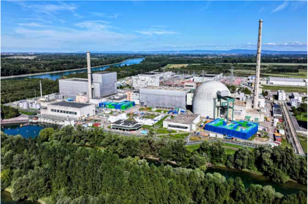
Figure 2-1 Aerial view of the Philippsburg plant complex (KKP 1 and KKP 2)
